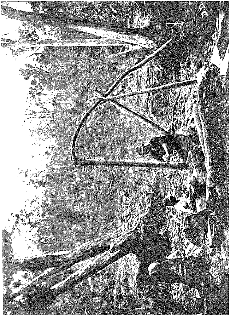
Pl: Crushing ore with a spring dolly [A.R. 1904]
