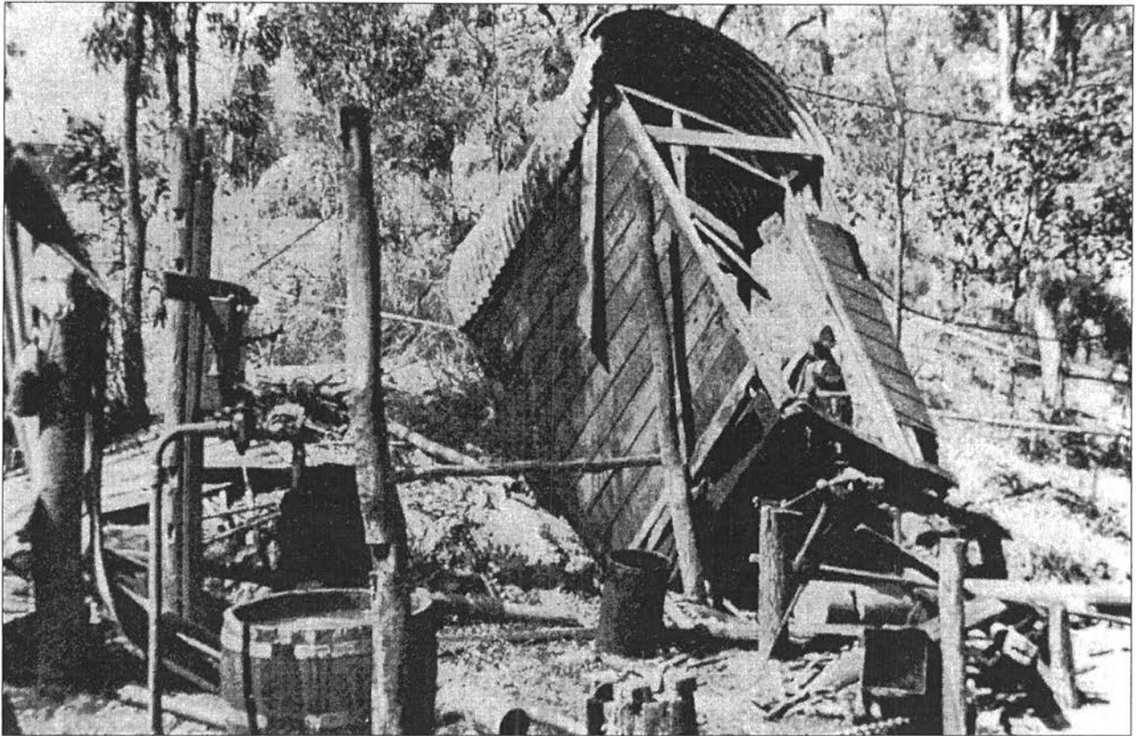
15. The Wrecked Blacksmith's Shop It stood outside the mine entrance near the junction box.
