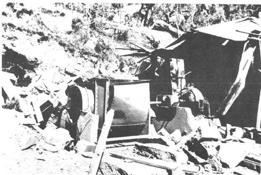
The ventilating fan motor, blown from the return airway (Number Three Tunnel) by the explosion. (Taylor/ Q.G.M.J. 15 October 1921, p.399)
