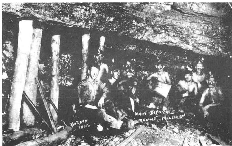
Miners in the underground workings about 1930. Note the timber props and stone packwall at left. (Kingdon/Jim McColm)
